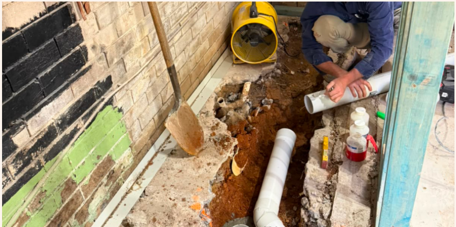
Excavation and new access point. A real KPD job, Northern Beaches.
